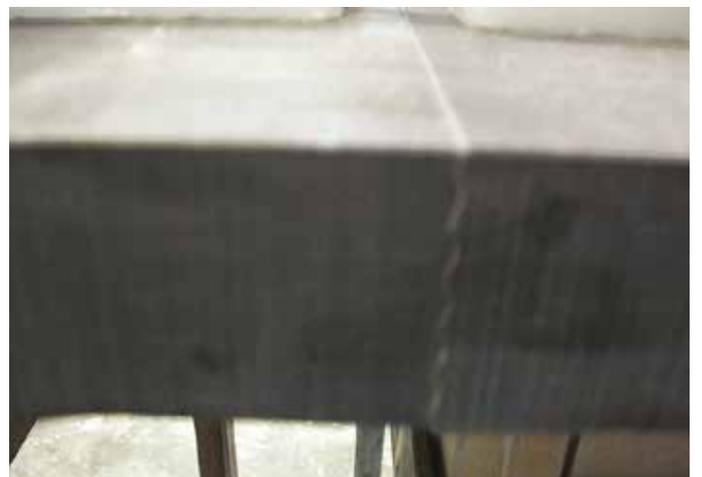
The use of a wavy bit for seaming is an excellent technique for aligning the panels and creating high resistance during the gluing procedure. However, specialised training and experience are essential. **If you do not have the necessary knowledge to use a wavy bit, we advise you to not use this technique on PaperStone®.**
