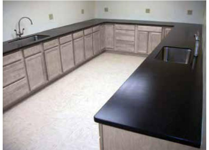
Kitchen and bathroom worktops must always be treated with Osmo® TopOil. The treatment must be carried out with a double application **on the top, bottom and edge of the countertop.**
